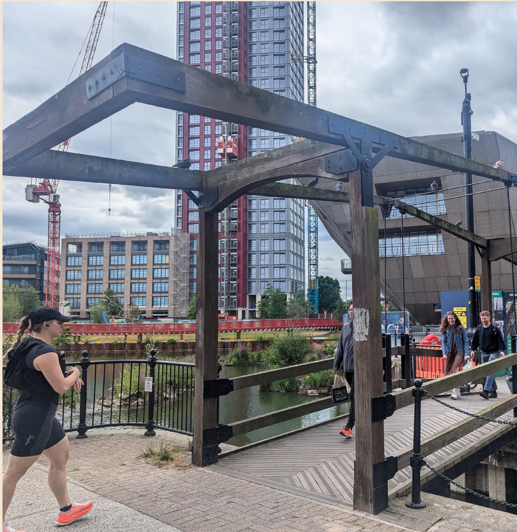
Existing view of Albion Bridge
