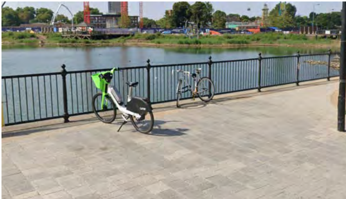
Existing metal balustrade
