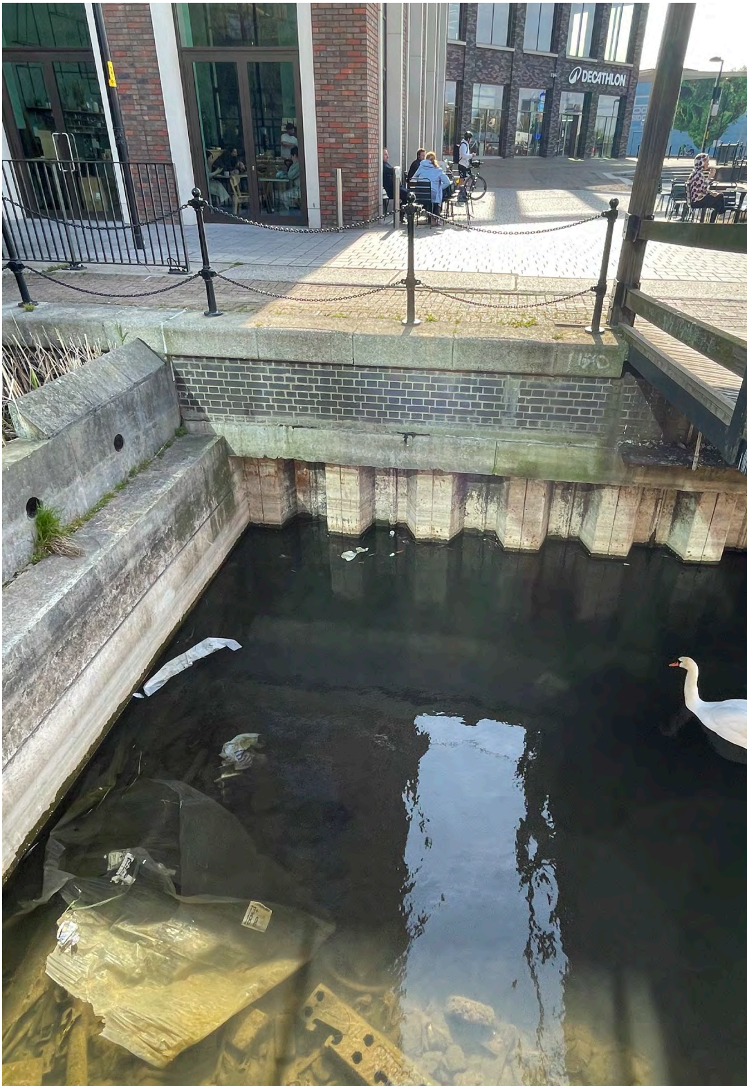
East side dock edge & Albion Channel weir/ dam
