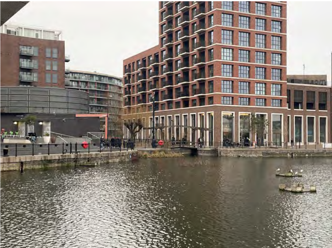
Existing timber footbridge - view from boardwalk
