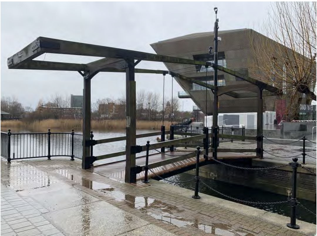
Existing timber footbridge - approaching from Albion Channel
