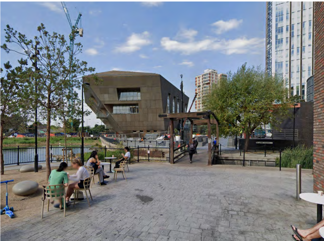
Existing timber footbridge - approaching from the west of Albion Channel
