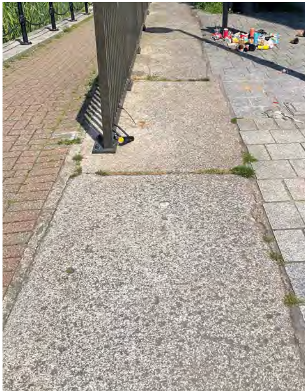
Existing historic granite dock edge slabs
