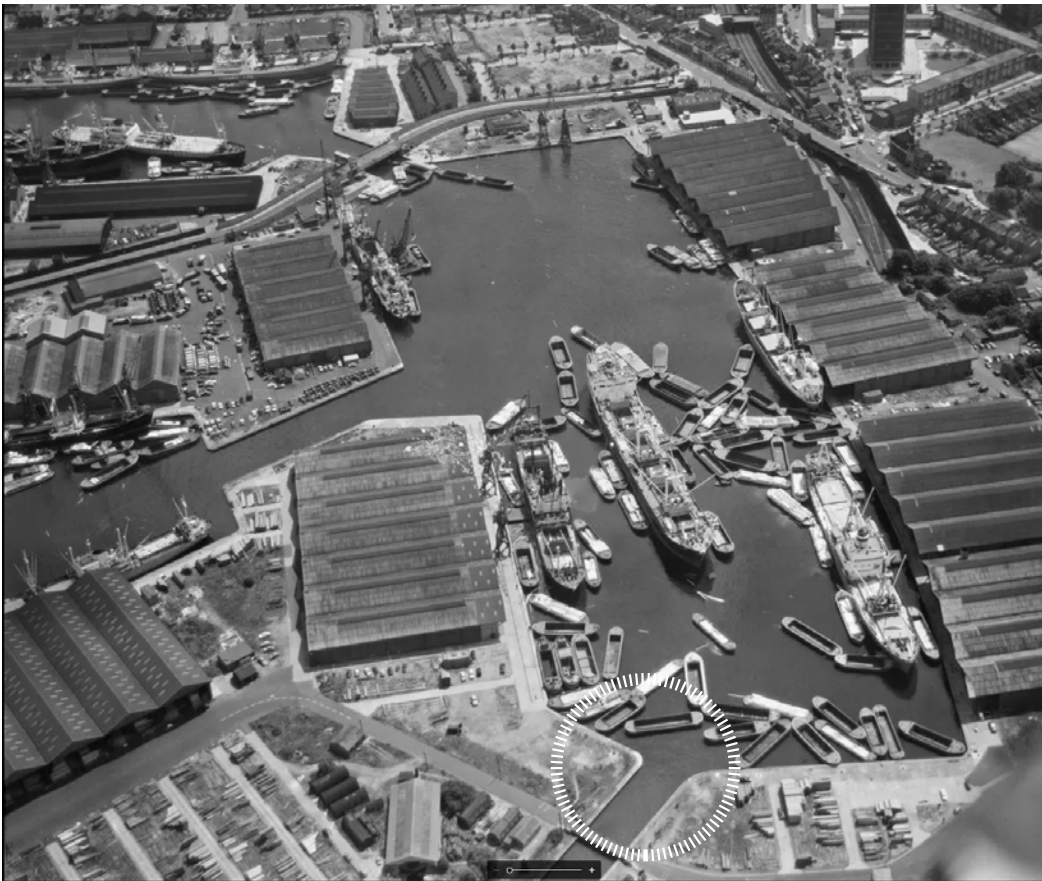
The highlighted area marks the original mouth connecting Canada Water Dock to the Albion Channel. Compared to the current opening, the historic photograph shows a significantly wider span between the two granite dock edges.
