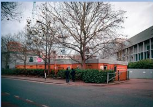
Southwark Construction Skills Centre
