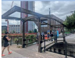
Albion Bridge - July 2024
