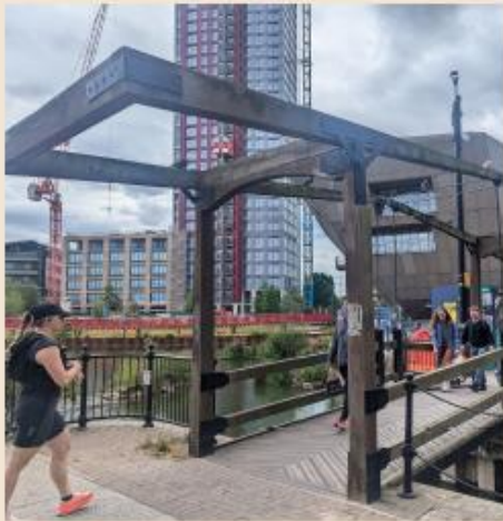
Existing view of Albion Bridge
