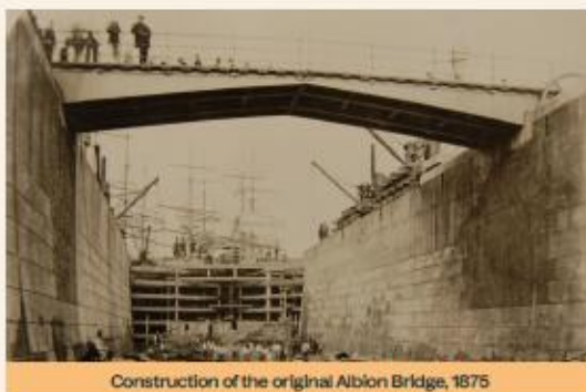
Construction of the original Albion Bridge, 1875
