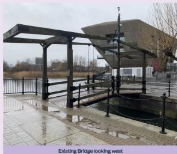
Existing Bridge looking west
